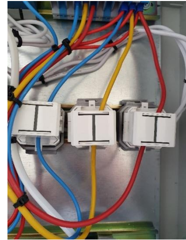
Fig. 5. Current transformers 120A
