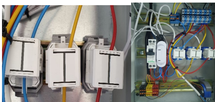
Fig. 4 - Sensor module mounting
